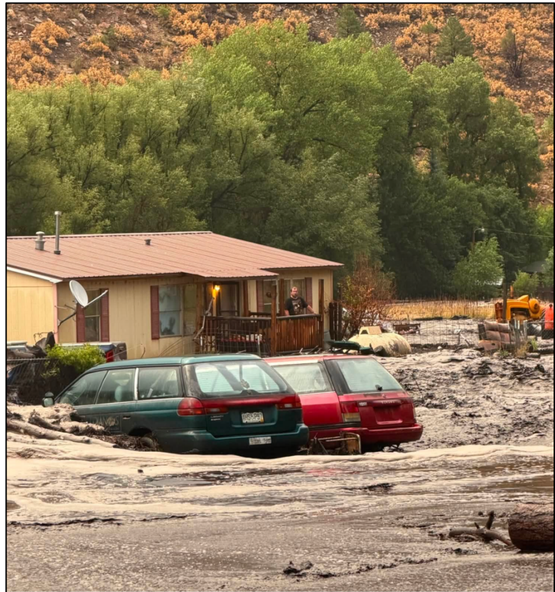
Figure 4. Damage from debris flow flash flooding in Beulah, CO on Jul 29, 2026. Photo credit: Pueblo County Sheriff's Office.
