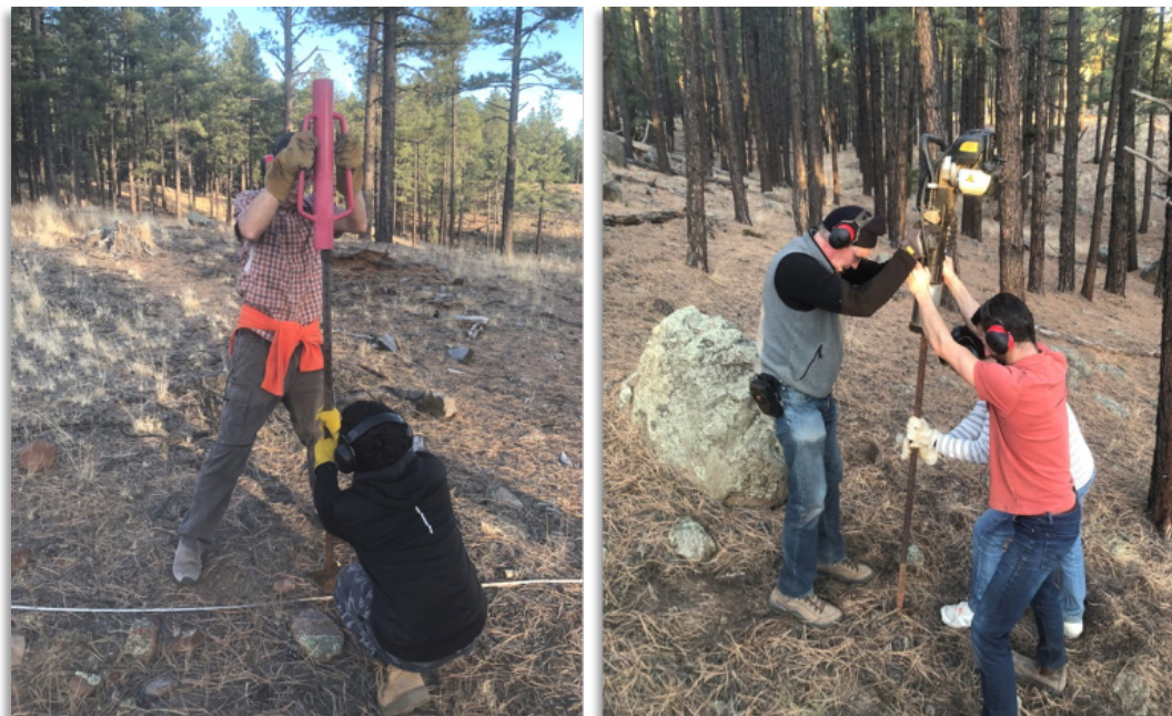
Figure 33. Driving T-posts into rocky soils near Flagstaff, AZ. Post location and rotation are first set with a manual post pounder, then a second team drives the post to the desired depth with a gas-powered driver. Photo: Joel Biederman.
